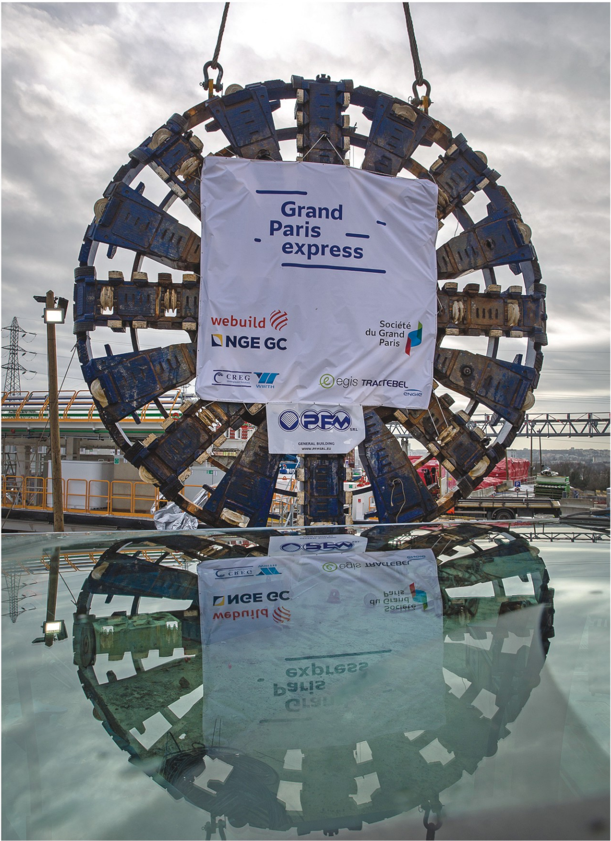
CREG TBM "Mireille" broke through on Line 16 of Grand Paris Express
