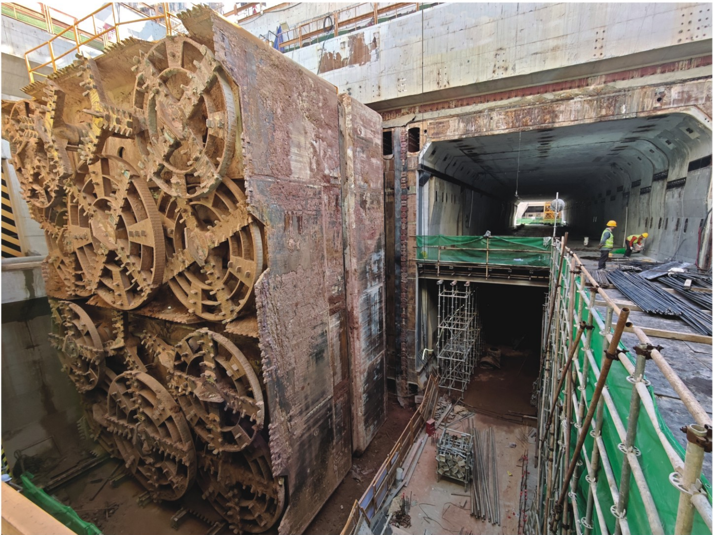
CREG TBM overcomes the challenge of ultra-small clearance excavation
