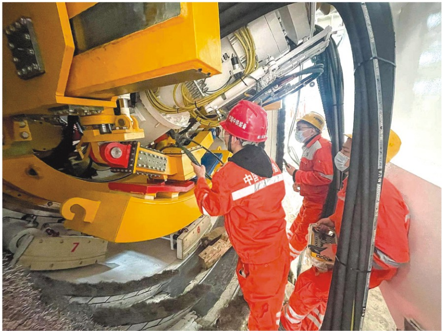
CREG service team at job site
