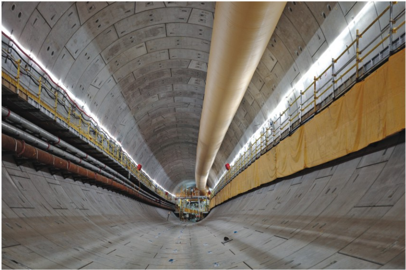
CREG's slurry collection system helps to create clean tunnel environment
