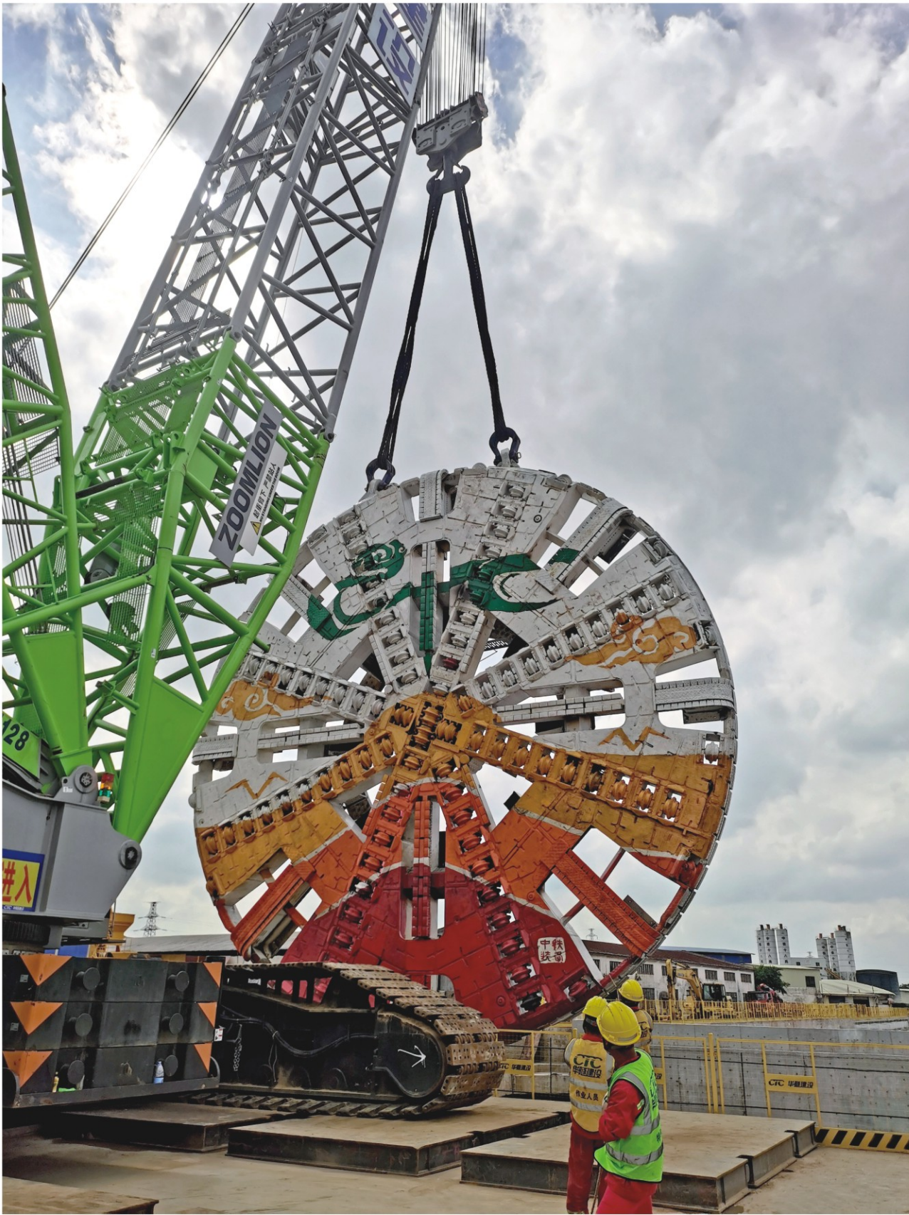
On-site assembly of the TBM
