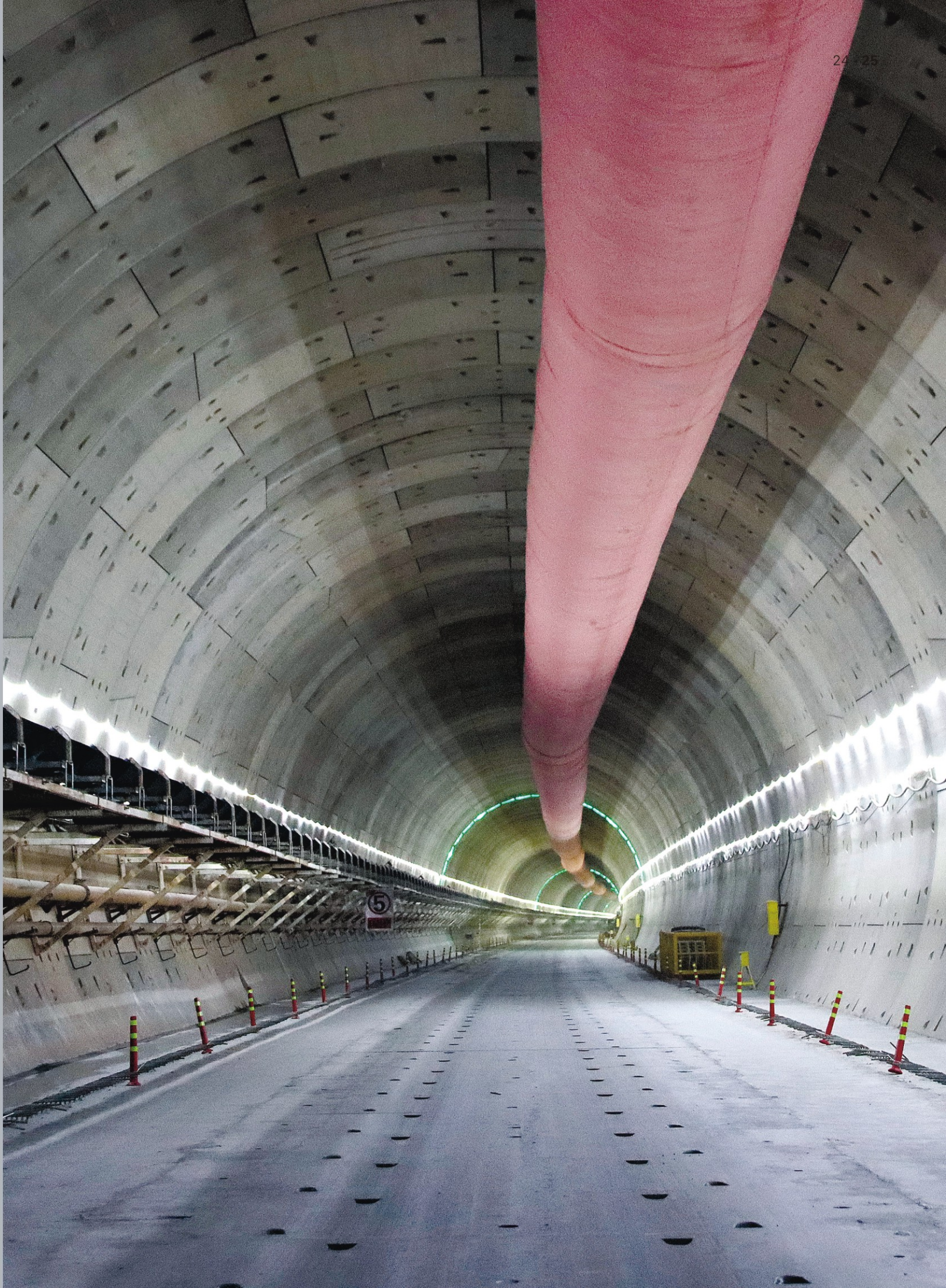
The \phi 14.29 m dual mode TBM has completed half of the 4.78 km long Guifeng Mountain tunnel of Zhuhai-Zhaoqing High-speed Railway, achieving a best monthly advance rate of 306 meters.
