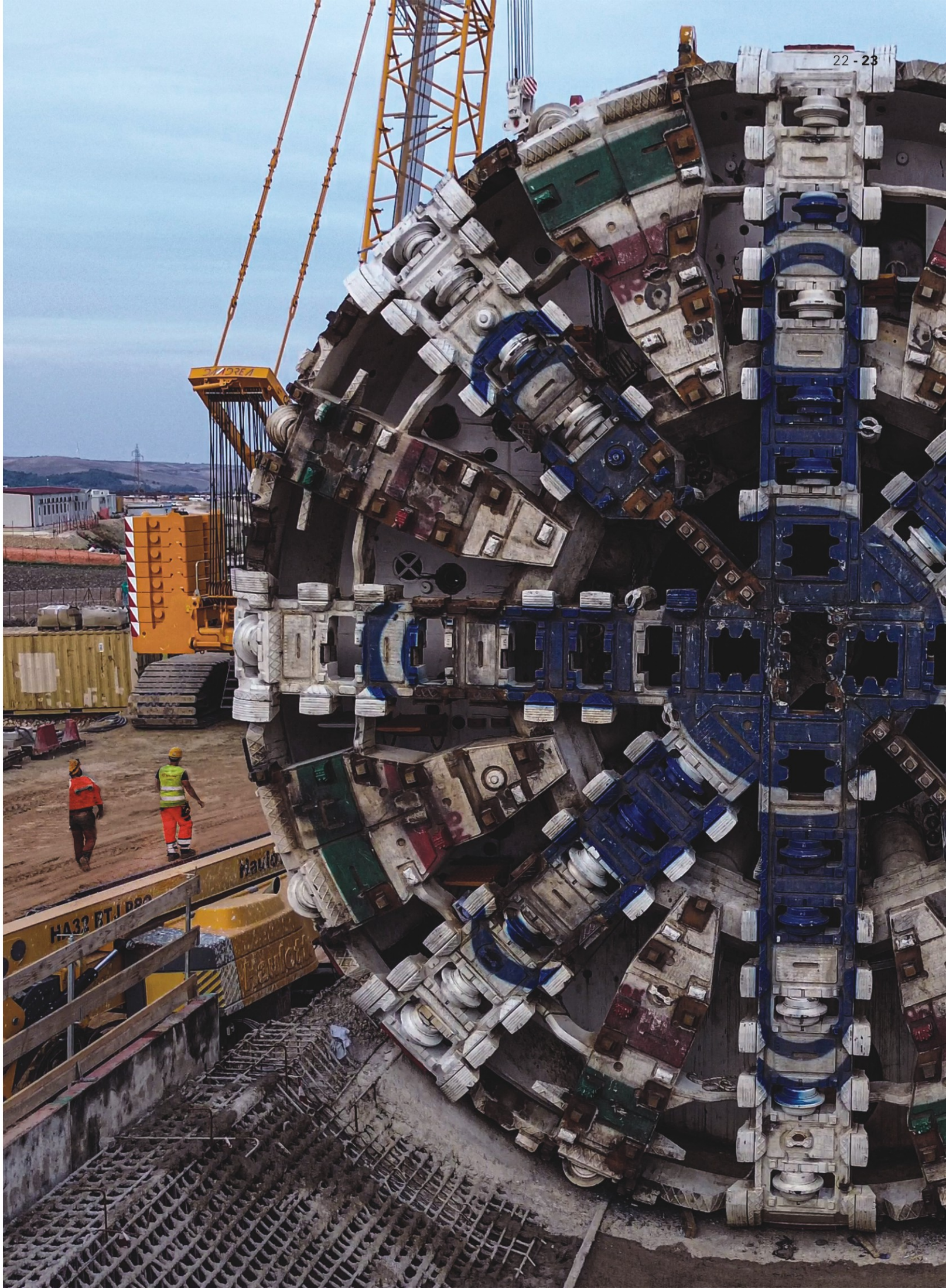
TBM assembly in progress for the Napoli-Bari Project in Italy.
