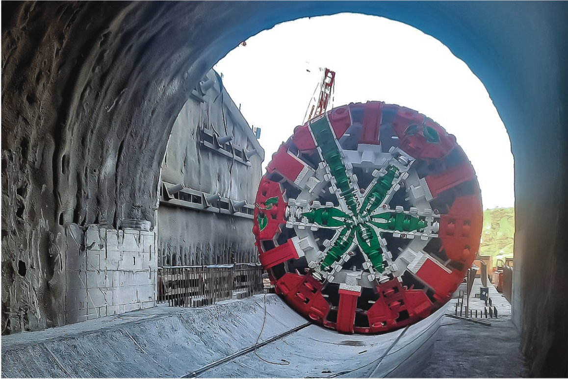
The green TBM starts the 10-km long travel through mountains.
