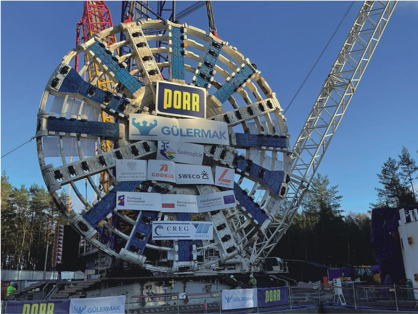
The cutterhead is being lowered down to the launching shaft
