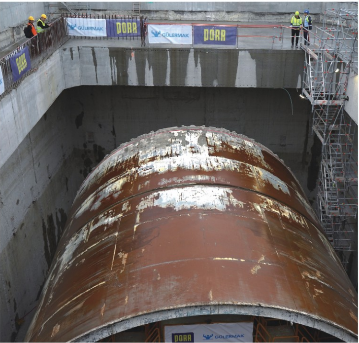
The large diameter TBM has overcome the challenge of 300 m radius curve.
