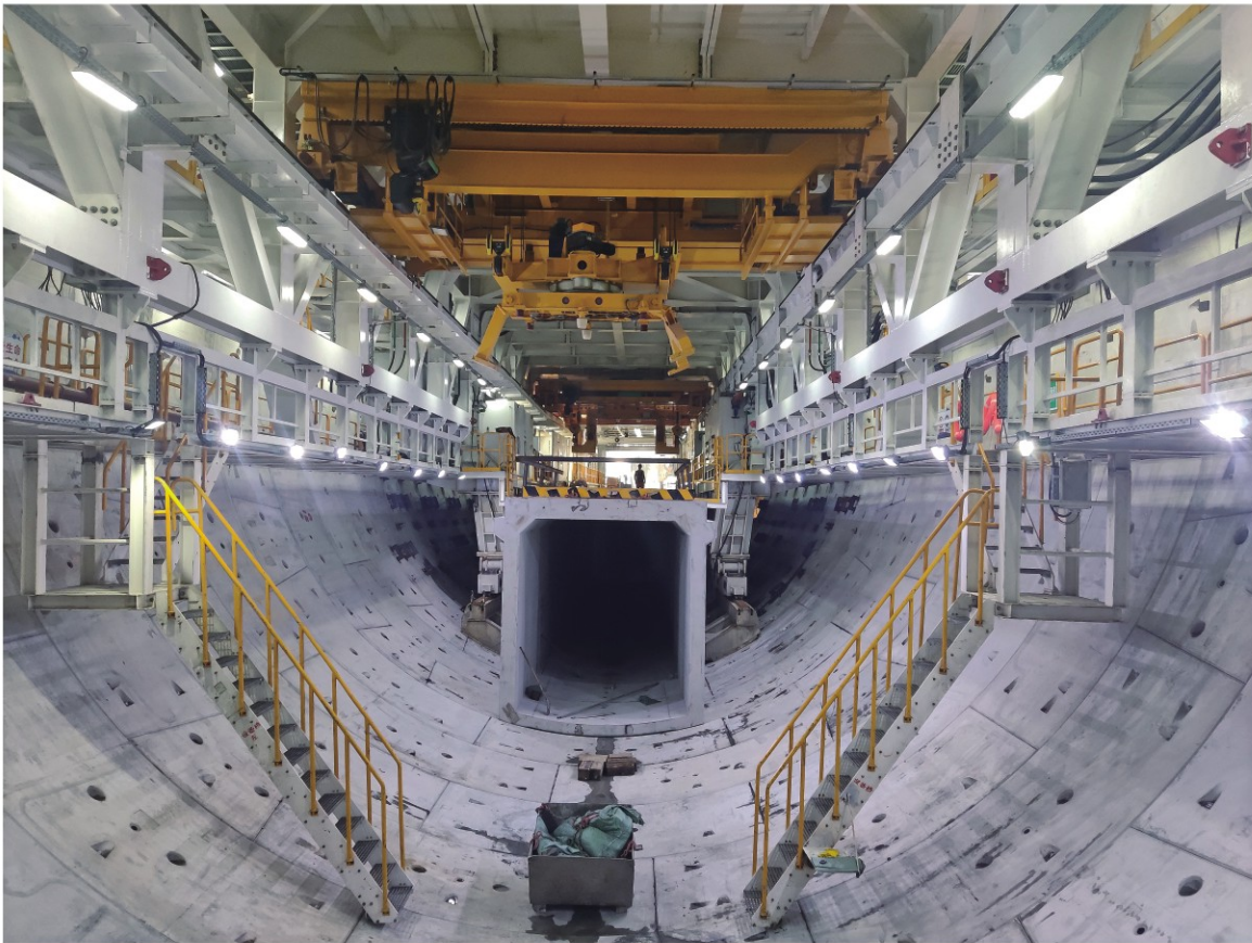
Box culverts are installed simultaneously as TBM advances.
