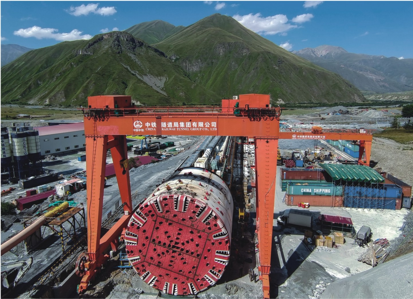
The TBM is ready to bore.
