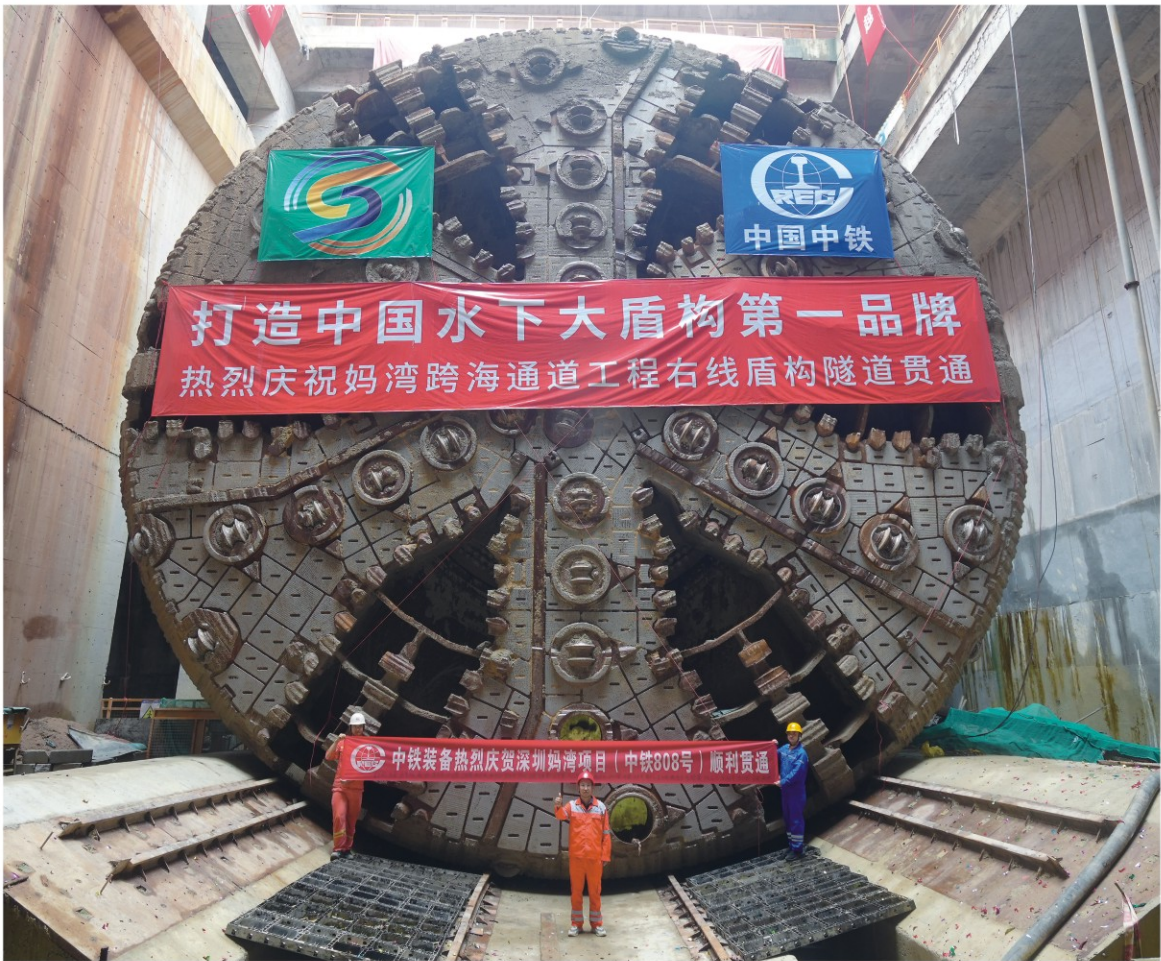
The TBM(CREC 808) has created a national record of 10 meters per day for large sub-sea TBM.
