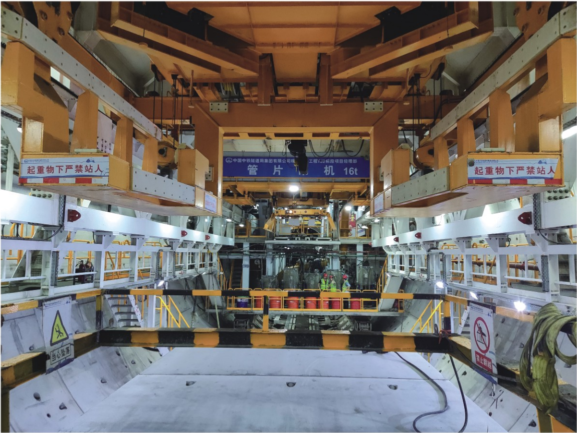
Box culverts are installed simultaneously as TBM advances.
