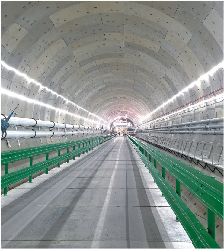
CREG slurry collection technology helps to create a clean tunnel environment.
