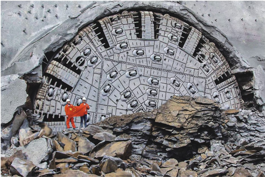
The "Caucasus" TBM completed tunnelling 30 days ahead of schedule.
