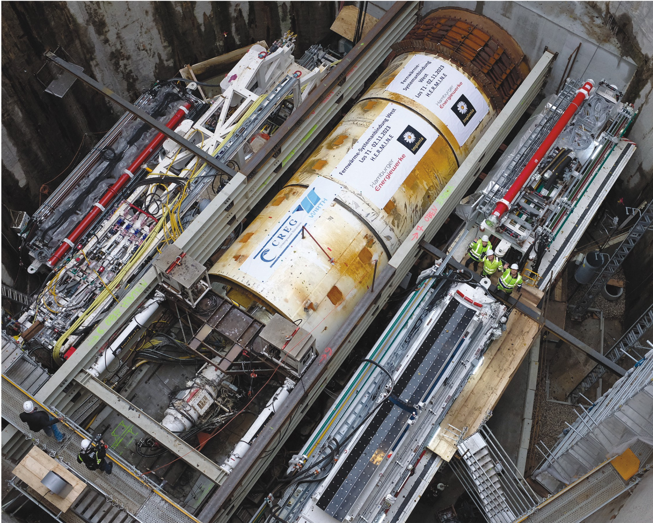
CREG has sent a service team to facilitate TBM umbilical launching in limited launching shaft.
