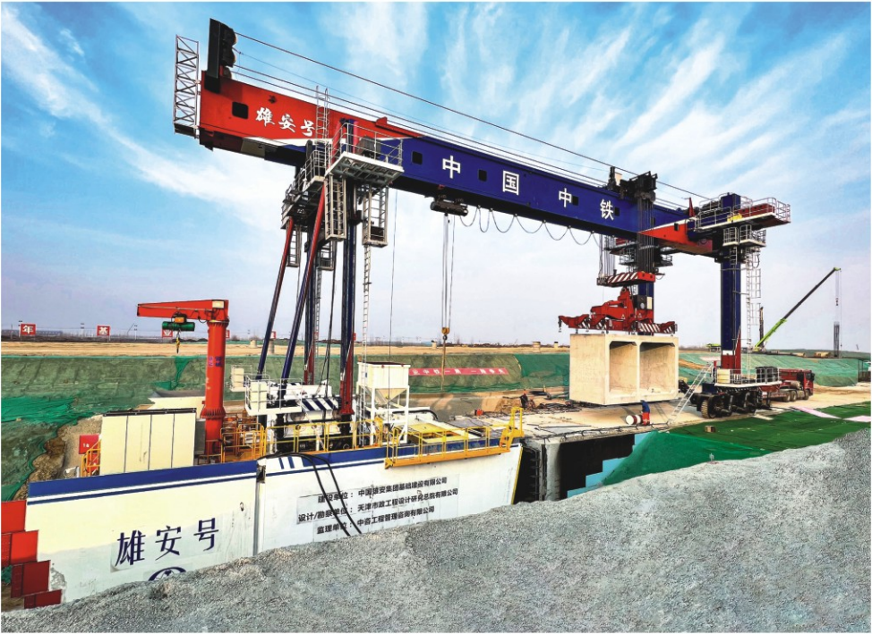
The project has created a new method of construction for open-cut tunnels.
