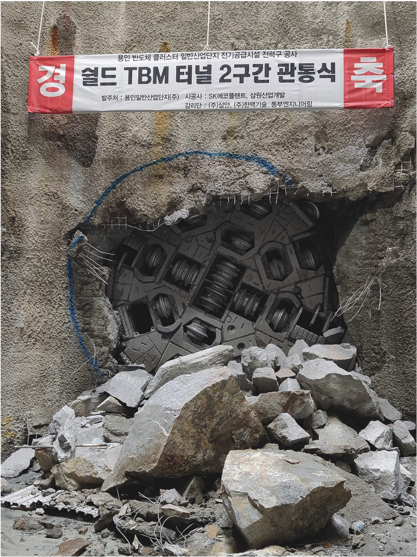
The TBMs completed tunnel breakthrough 7 months ahead of schedule with reliable performance.
