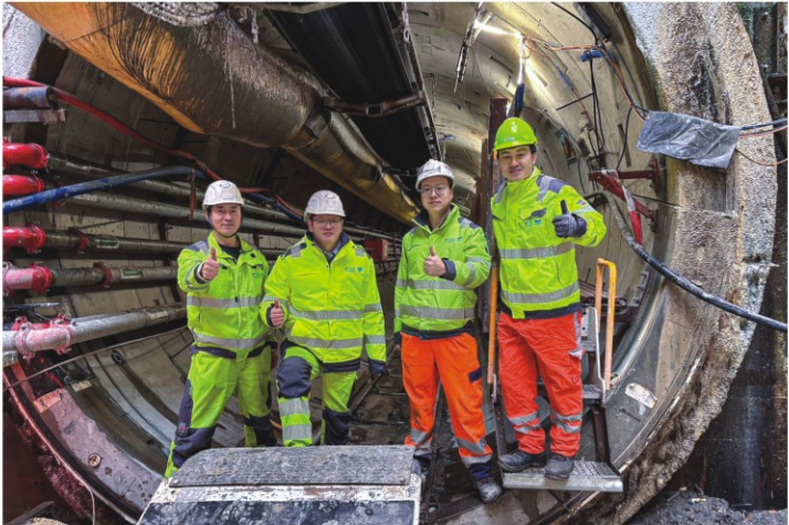
CREG service team celebrates the breakthrough of the tunnel.
