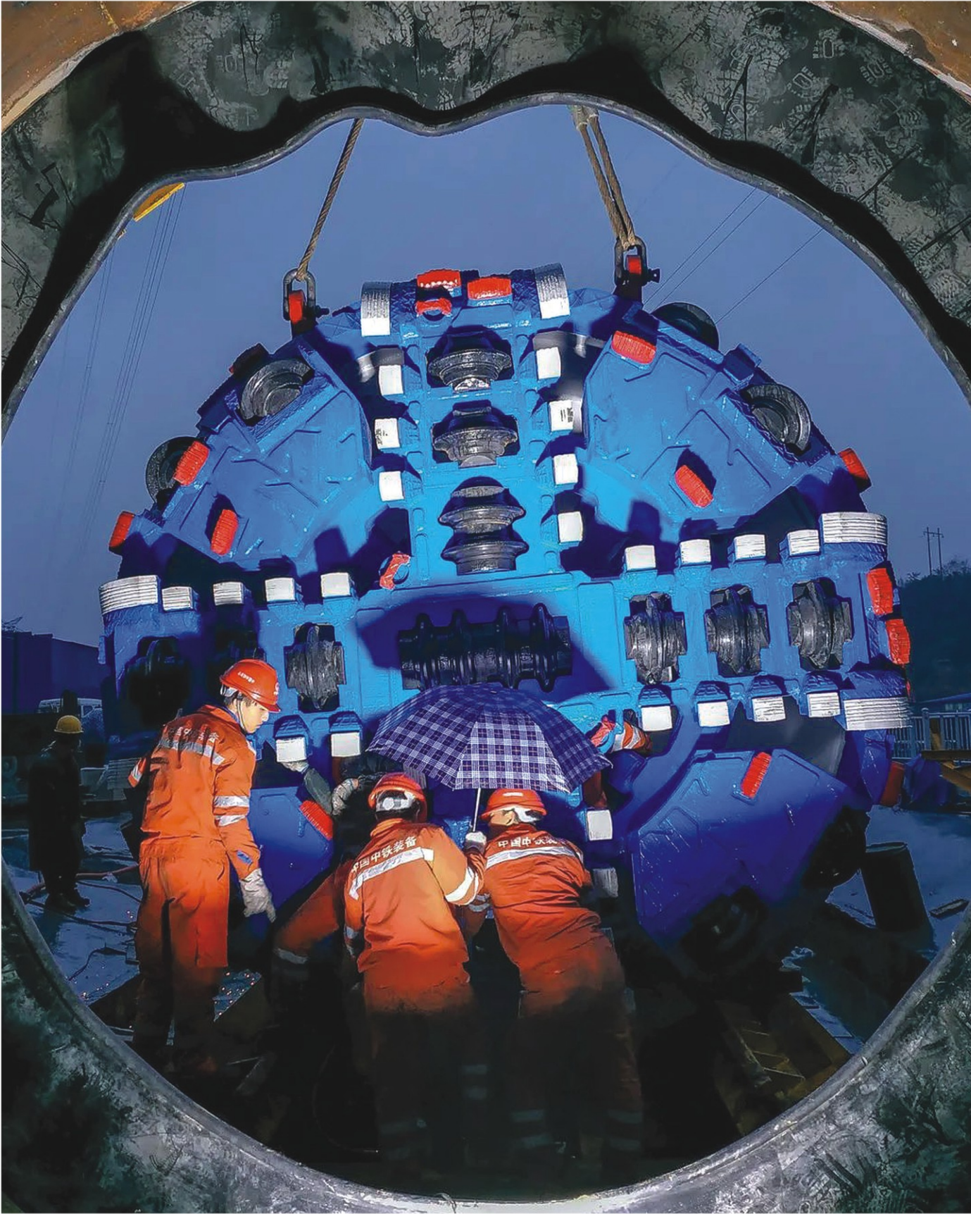
CREG service team is busy with TBM commissioning before launching.
