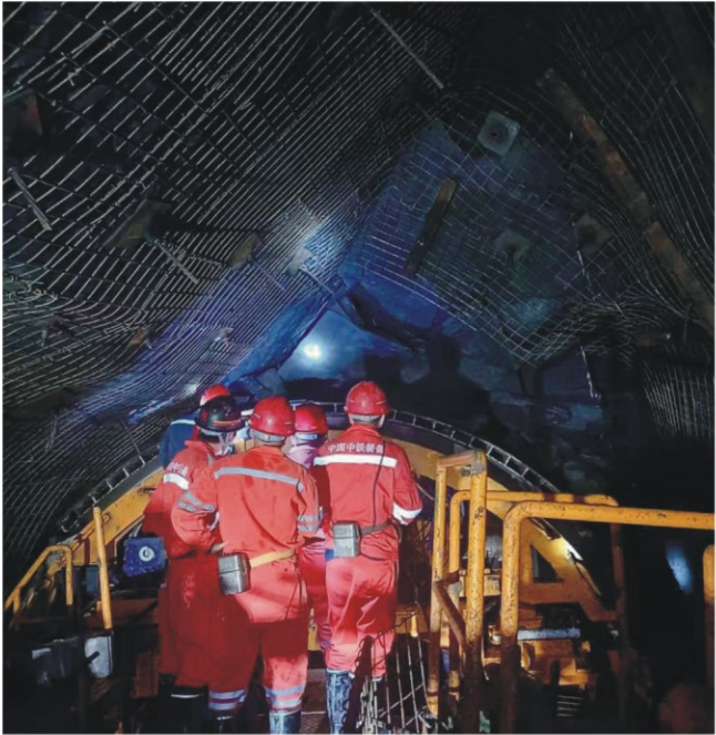
CREG has sent a technical service team to facilitate the TBM operation.
