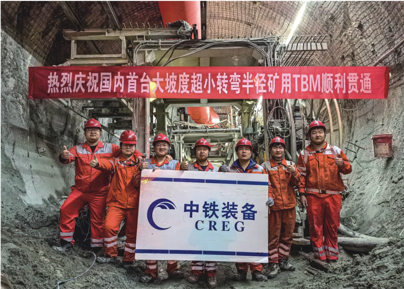
The TBM achieved tunnel breakthrough, boring over 500 m in a month.
