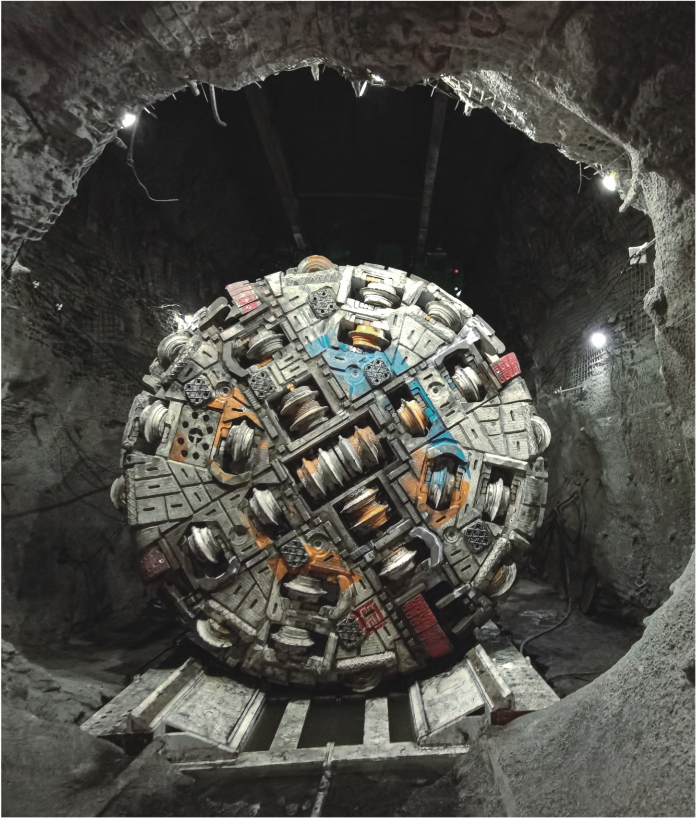
The TBM is ready to bore a 15 km long tunnel with a maximum overburden of 760 m.
