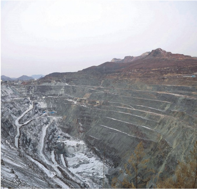
Construction of the roadway faces challenges of high ground temperature and large overburden.
