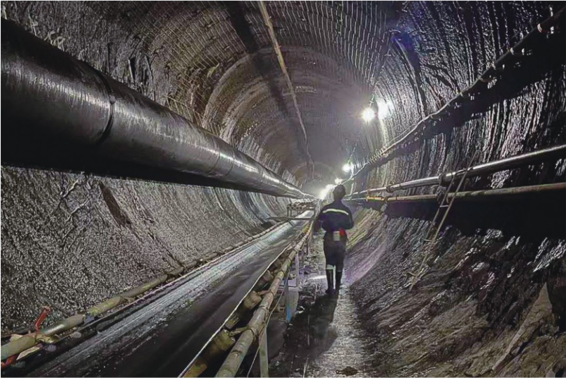
TBM method is able to build roadways efficiently in spite of the occurrence of caves and high content of gas and water.
