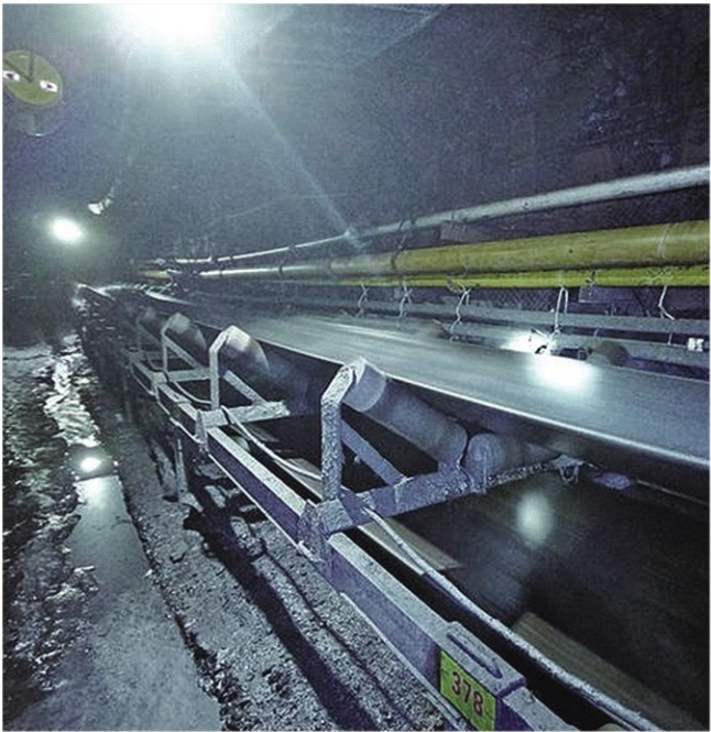
With the help of belt conveyor for rapid muck removal, the TBM bores 16 m one day.
