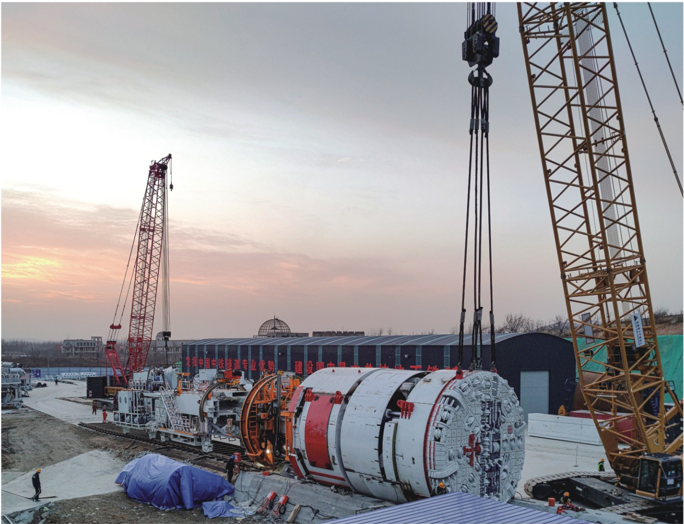
The TBM assembly is in progress. Once ready, it will bore a 10.5 km long tunnel, 6.3 km long with 15% downhill and 4.2 km long with 22.5% uphill.
