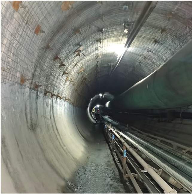
The TBM is boring steadily, advancing over 600 m in a month.
