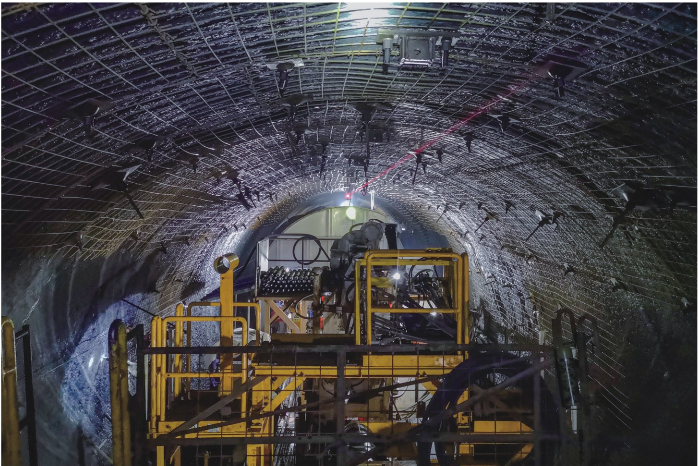
Advanced technologies enable the TBM to cope with complex working conditions.
