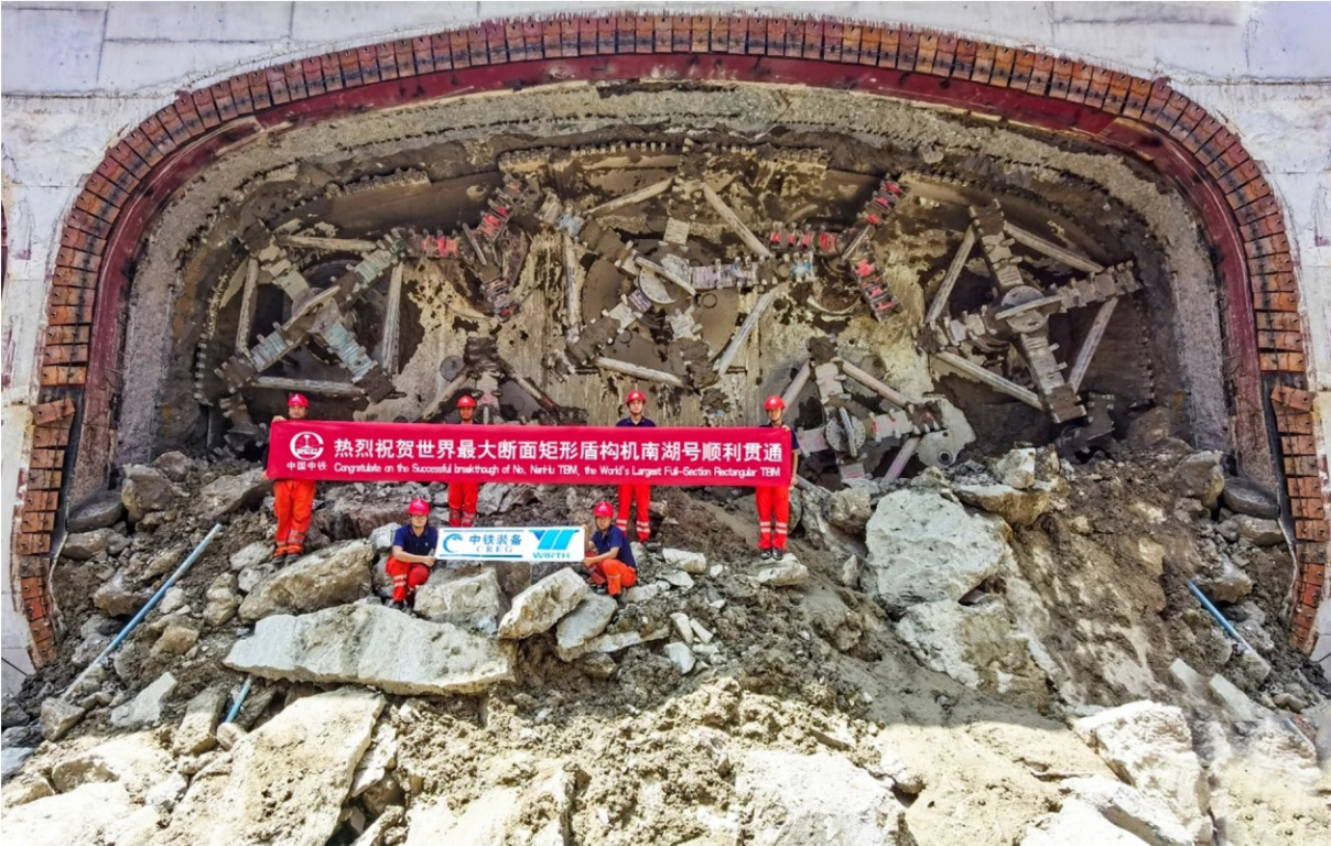
Successful breakthrough of the super-large cross-section rectangular pipe jacking machine.
