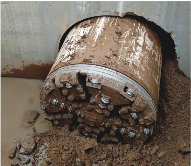
Large-section pipe jacking machine broke through.
