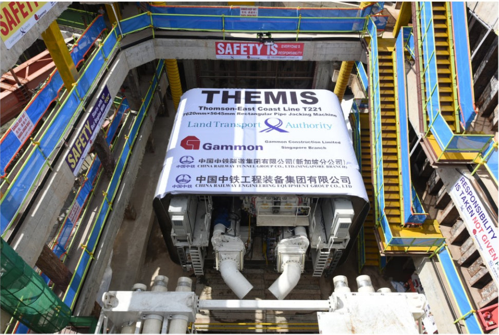
Launch preparation for the rectangular pipe jacking machine.
