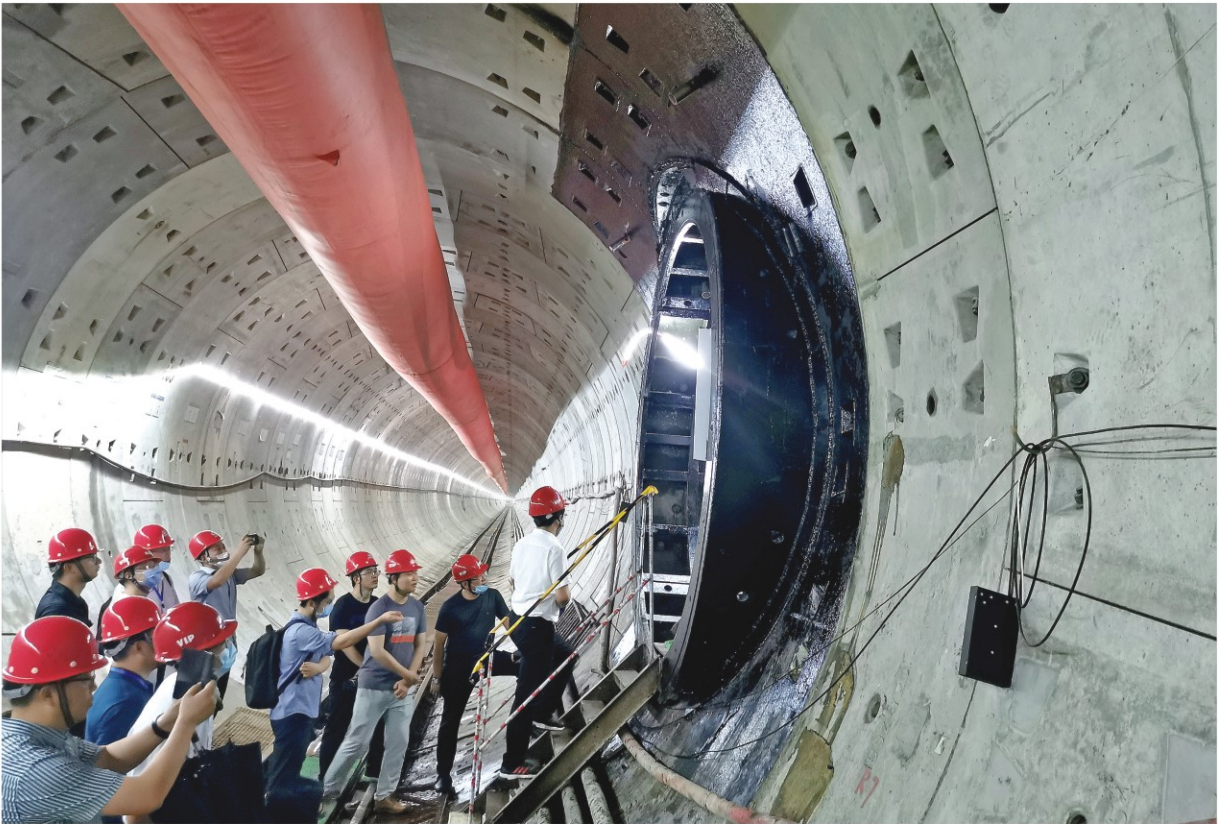
It creates a new construction method for metro cross passages.
