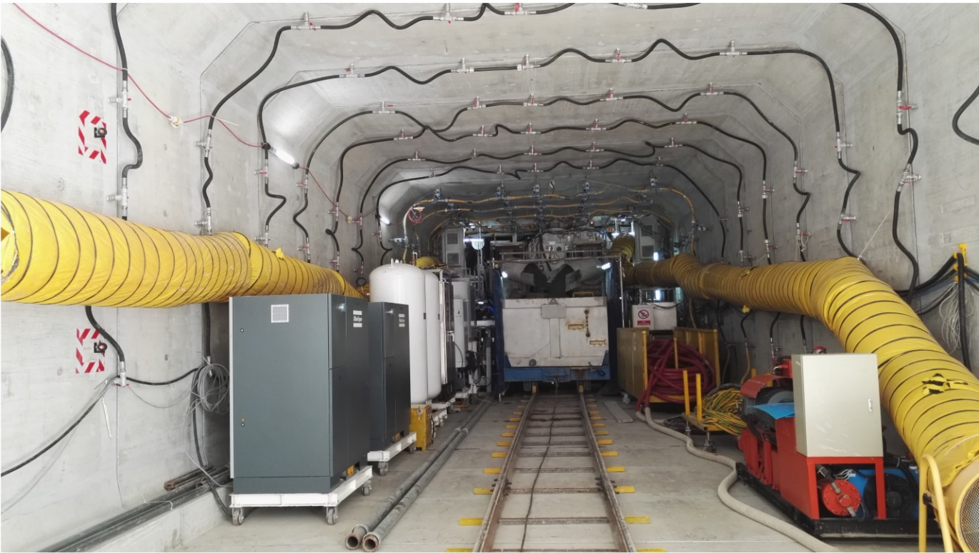
The project implemented standardized management and was awarded the Singapore Project Management Gold Award in 2016.
