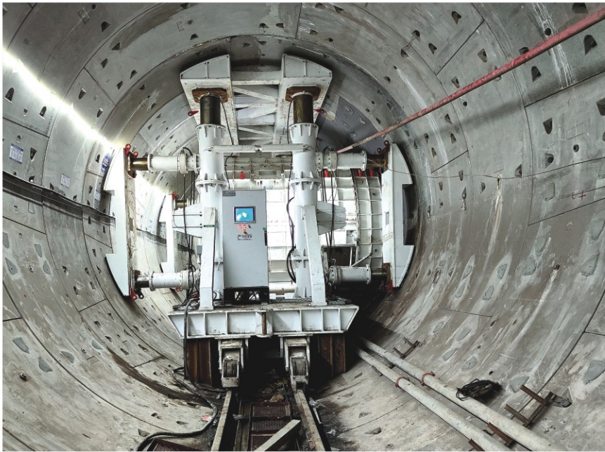
Machine construction in a formed metro tunnel.
