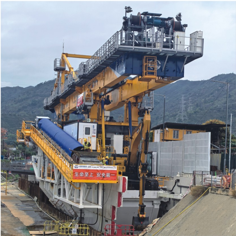
The project has created a new method of construction for open-cut tunnels.
