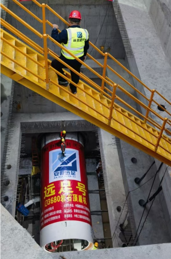
The pipe jacking shield machine meets the needs of long-distance municipal pipe gallery excavation.
