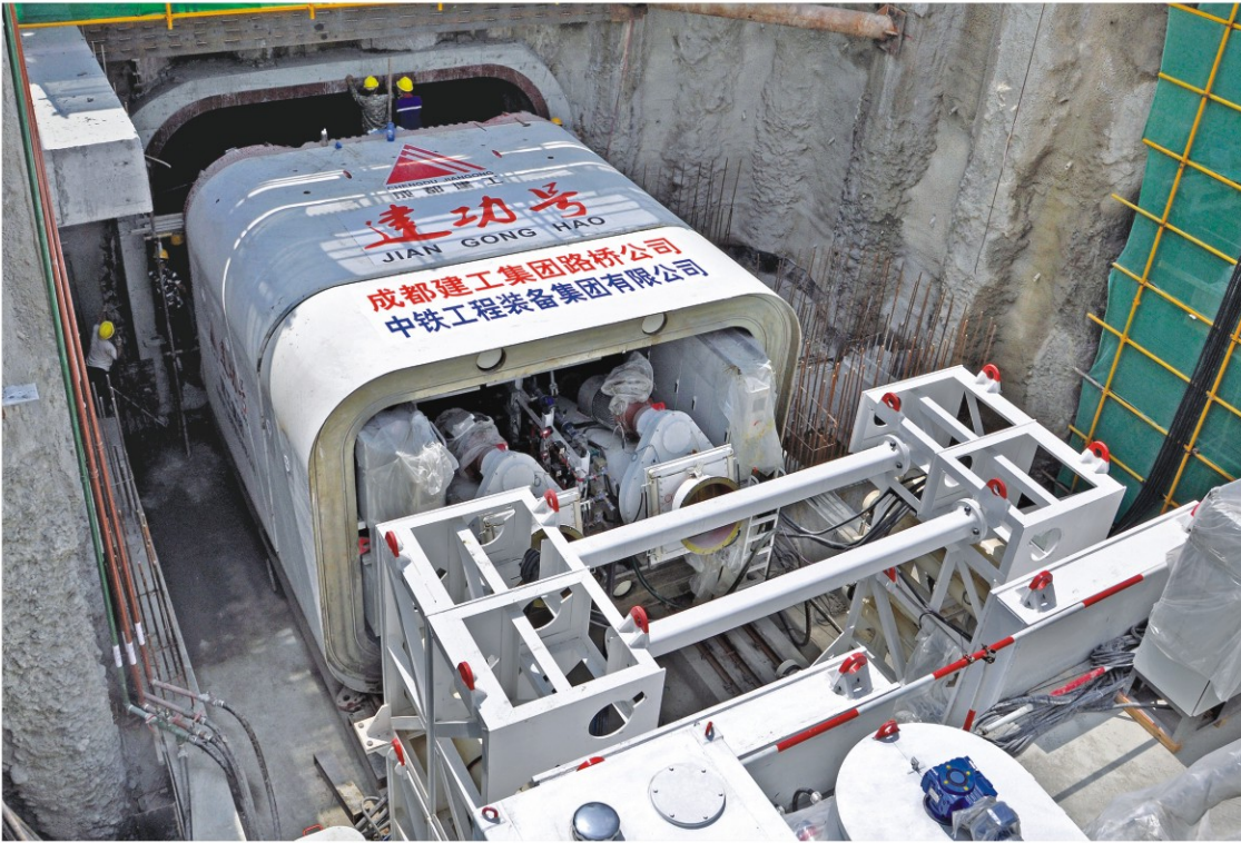
Machine is entering sandy gravel strata for construction.
