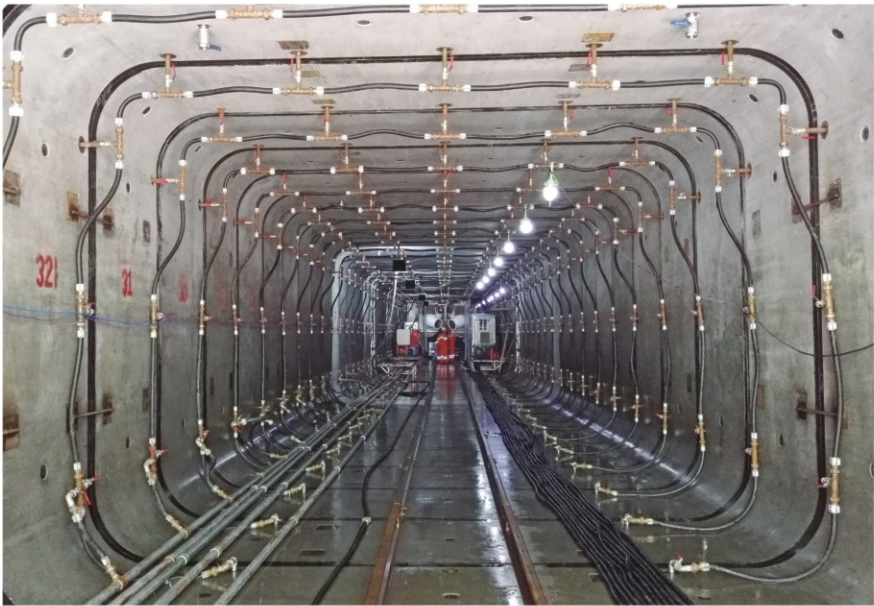
Tunnel after completion.
